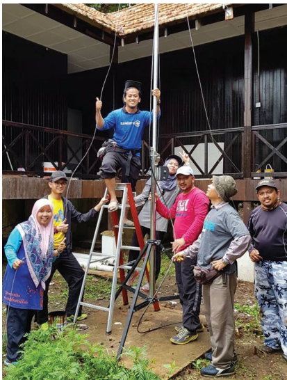
Figure 3. On-site Yagi antenna installation.
