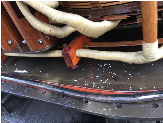
FIGURE 10. Scene picture: metal particles in the oil.
