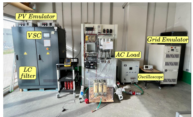
FIGURE 5. Test bed implemented.
