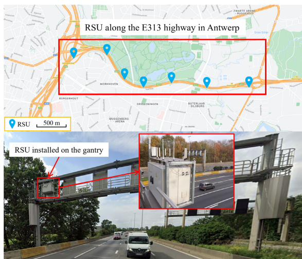
FIGURE 4. RSUs deployment along the E313 highway in Antwerp (upper) and RSU used for measurements and its installation position on the top of a gantry (lower).
