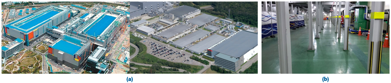
FIGURE 2. Fabs and columns: (a) Aerial views of fabs. (b) Columns in the indoor environment of a fab under construction.
