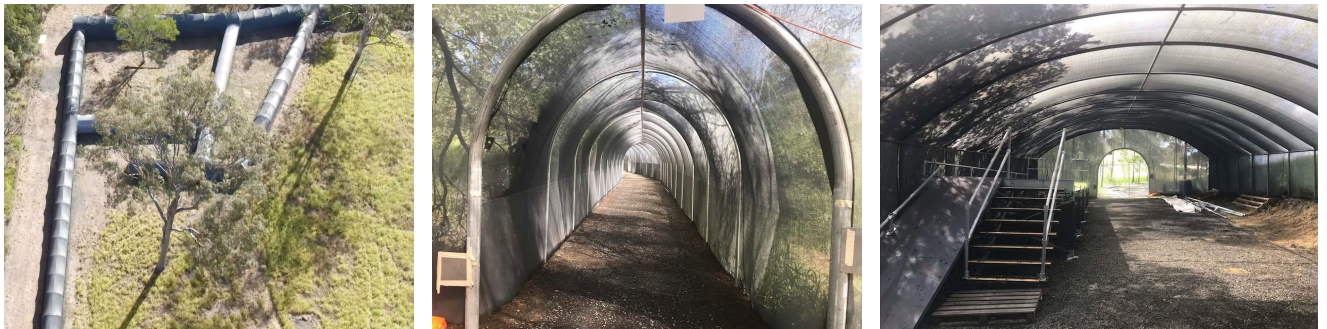
FIGURE 17. Aerial view of the shade-cloth tunnel with an overall length of over 300 m built at CSIRO’s QCAT site in Pullenvale, QLD, Australia (left), an inside view (center), and stairs and mezzanines built inside the tunnel (right).
