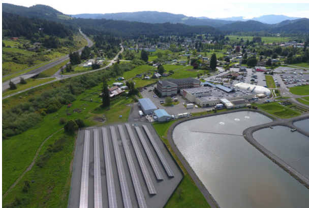
Fig. 4 Overview of the BLR community microgrid (Source: Schatz Energy Research Center, Humboldt State University) [31] .
