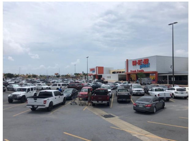
Fig. 5 Grocery store in Texas that retained power supply by a microgrid during the winter storm (Source: Courtesy of Enchanted Rock) [33] .
