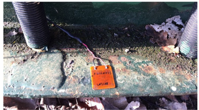
Fig. 12. Attached FSM transducer on the 4 m diameter tank floor without any surface preparation.
