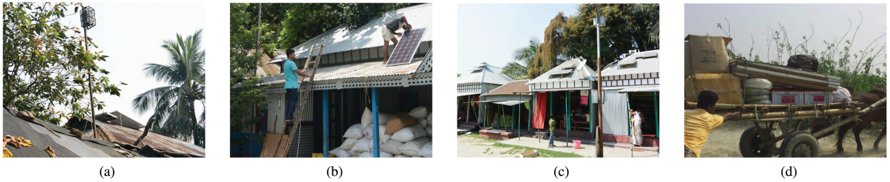
Fig. 5. Examples of practical realizations of the three design features as observed in various swarm microgrids in Bangladesh. (a) Self-serviceability: Communication tower containing a wireless local area network router. (b) Self-serviceability: Adaptations being made to a swarm microgrid in operation. (c) Sustainability: Several shops with solar panels, illustrating the usage of 100% renewable energy. (d) Scalability: Additional components being brought to a site for modular expansion of the swarm microgrid.
