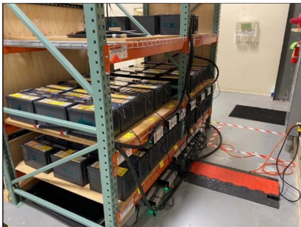
FIGURE 7. VRLA battery bank used in experiments performed at EPRI.
