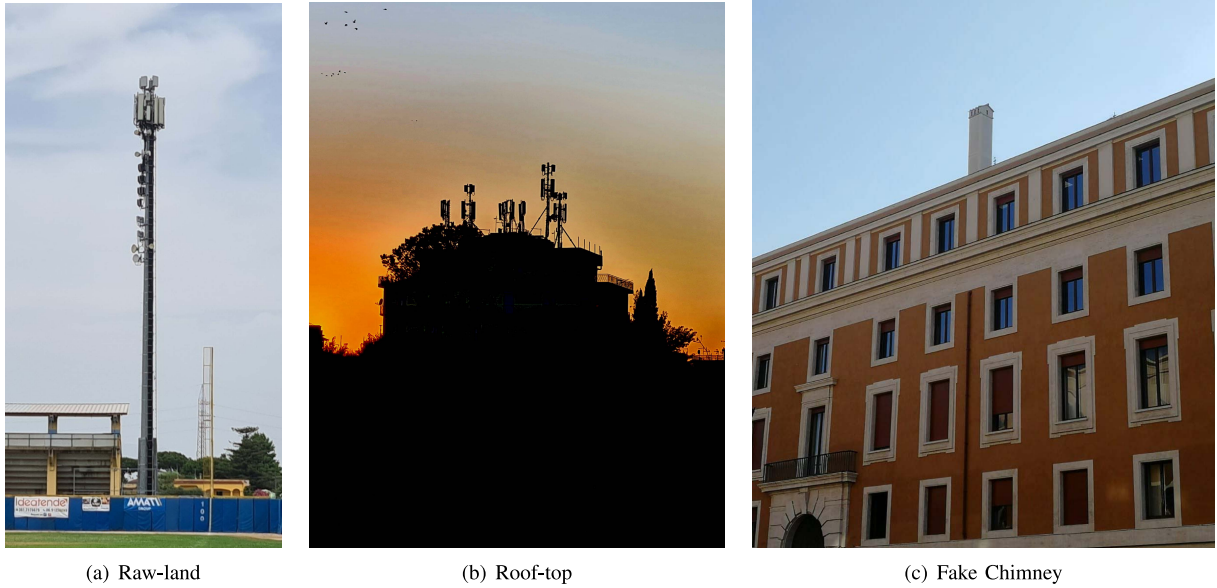
FIGURE 4. Main types of cellular towers.
