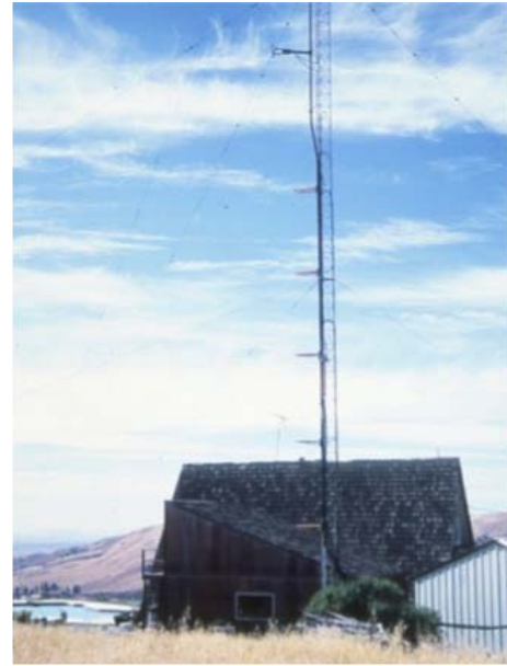
FIGURE 15. House close to a radio broadcasting tower in San Jose - CA (photo by Richard A. Tell). The EMF field measured in the proximity of the house was higher than 61.4 [V/m].
