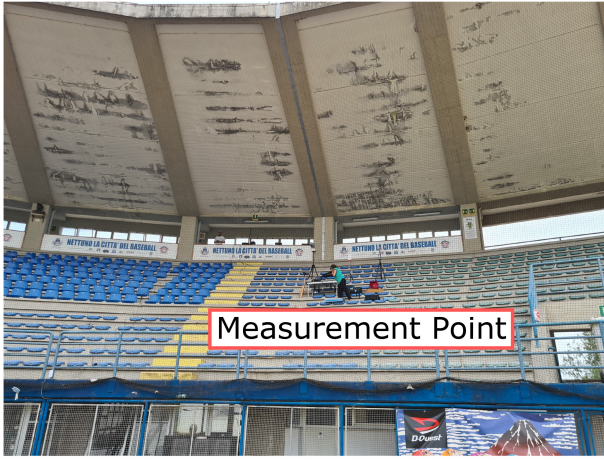
(a) Field view of the measurement point.
