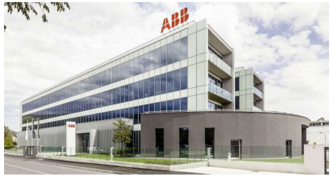
Fig. 1. ABB office building whose electric load consumption has been collected in dataset A.
