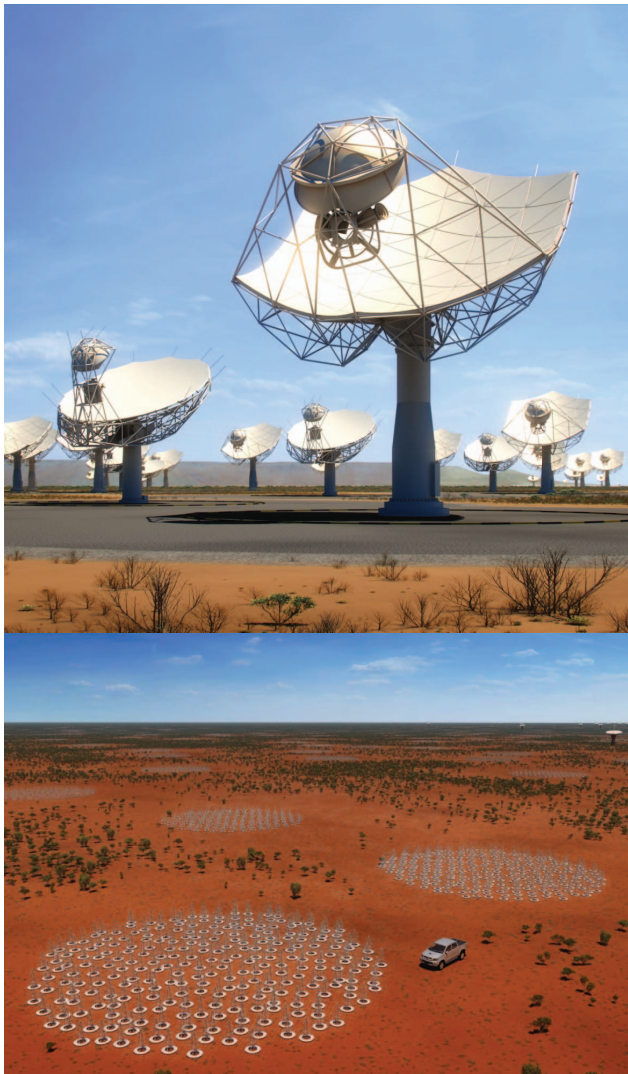
Fig. 1. Top: Dishes for SKA-Mid, in South Africa, will generate 62 exabytes of raw data per year – enough to fill 340,000 average laptops with content every day. Bottom: Aperture arrays for SKA-Low, in Australia, will generate 5 zettabytes of data per year. Unlike conventional dishes, the “beam” of these antennas can be formed electronically – allowing each antenna to look at multiple regions of the sky simultaneously. The total field of view is essentially limited by the signal processing capacity. Image Credits: SKA Organisation.
