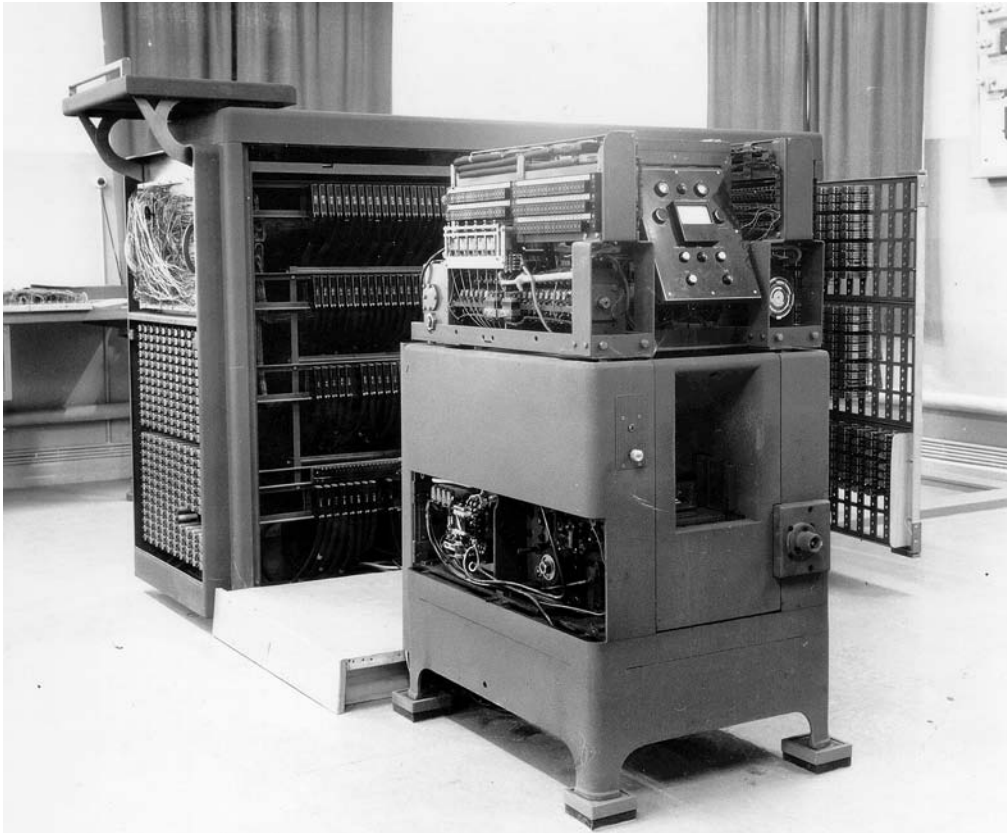
Figure 2. Zuse's electromechanical calculating punch M9 mass-produced in cooperation with Remington Rand, Zurich (courtesy of Max Forrer).
