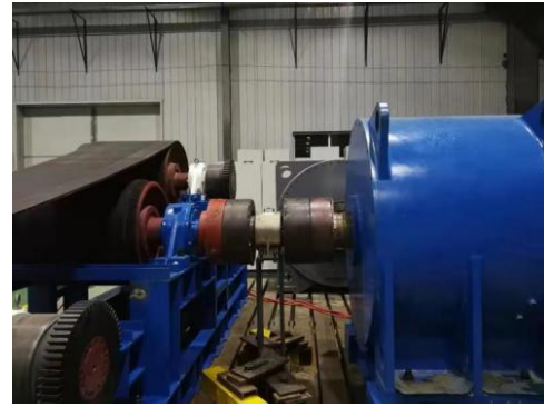
Fig. 16. Temperature rise experiment platform.
