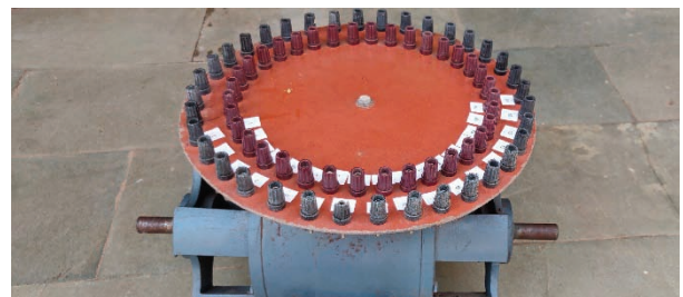
Fig. 12 Rewinding process for the motor winding and testing the tappings, done on the stator coils of Phase-C
