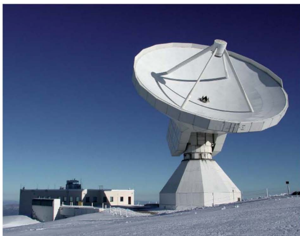
Figure 12. The 30-m millimeter radio telescope (MRT) of IRAM at 2850 m altitude in the Sierra Nevada of southern Spain. Completely wrapped in thermal insulation and with active control of the temperature of the structure, it operates down to a wavelength of 0.8 mm (J. Baars, IRAM).
