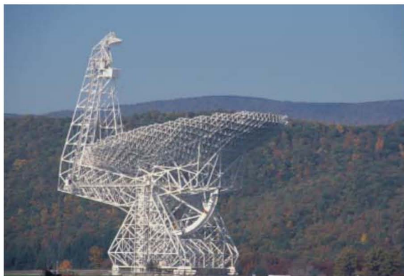
Figure 10. The Green Bank Telescope is an offset paraboloid of 100 m diameter. The reflector is actively adjusted to the correct shape by motorized adjusters on the basis of computed gravitational deformation. An overall surface error of 0.4 mm has been achieved (NSF/AUI/NRAO).
