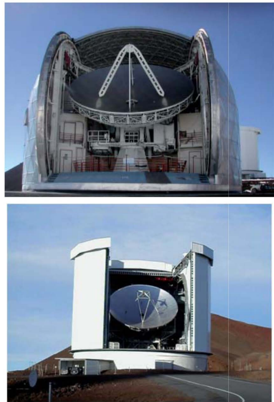
Figure 23. Two sub-millimeter telescopes at 4000 m altitude on Mauna Kea, Hawaii. (a) The Caltech telescope, with a diameter of 10.4 m, operating at a shortest wavelength of 350 \mu\text{m} (S. Golwala, Caltech). (b) The JCMT with a diameter of 15 m, normally protected by a transparent skin covering the enclosure opening. Observations are made at wavelengths between 0.4 mm and 1.4 mm (Phillips, JCMT, Hawaii).
