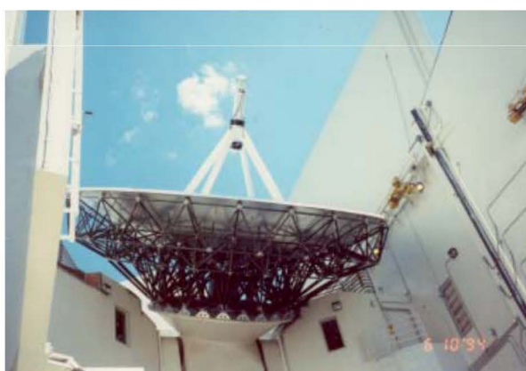
Figure 24. The HHT sub-millimeter telescope in the opened enclosure at 3200 m altitude on Mt. Graham, Arizona. The truss frame backup structure (black) consists of carbon-fiber-reinforced plastic struts connected to invar steel nodes. The connection to the steel elevation structure (white) is made by 20 flexures of steel. These effectively absorb the difference in thermal expansion between backup and mount without introducing deformation into the backup structure (J. Baars, SMT Observatory).
