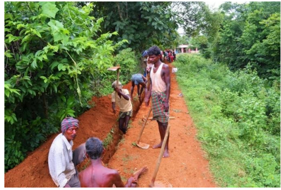
Fig.8: Community participation in trench digging
