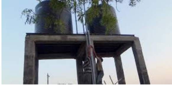
Fig.6: Storage Tank and Structure in Harirampur
