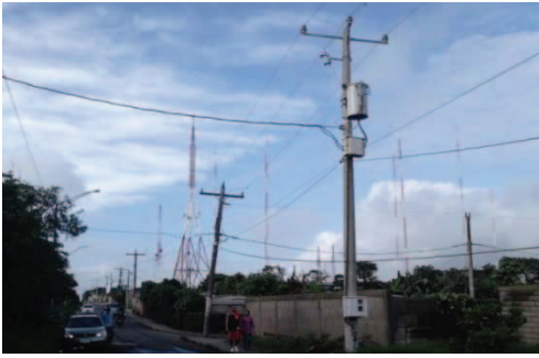
Fig. 2. Some FM Radio and TV transmission systems visualized near houses in El Crucero.
