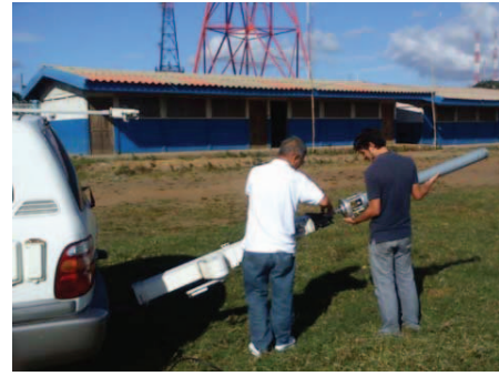
Fig. 10. Installing the HE 309 antenna to the mast.
