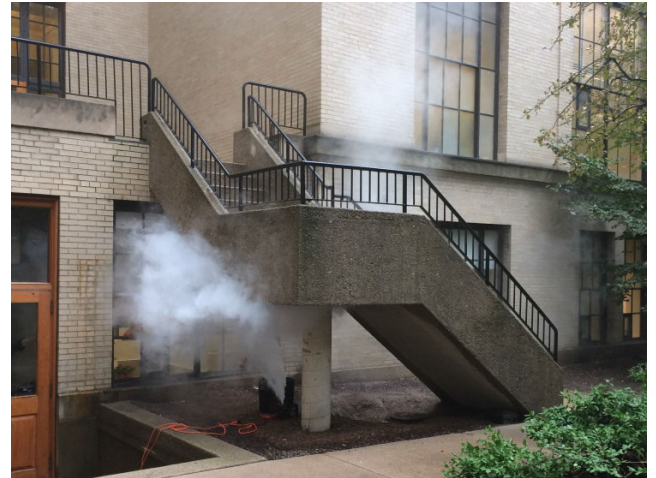
FIGURE 14. Small scale test showing destruction of DC link capacitors.
