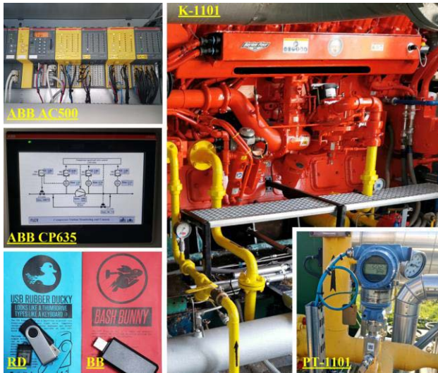
FIGURE 5. Compressor station parameter alteration during LCSA attack (top), and real process/experimental equipment (bottom).
