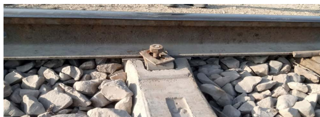
FIGURE 13. Loosed nut bolts.
