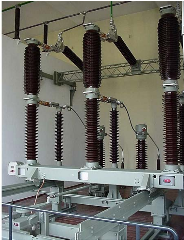
FIGURE 24. LTB-D high voltage Live-Tank circuit breaker by ABB.
