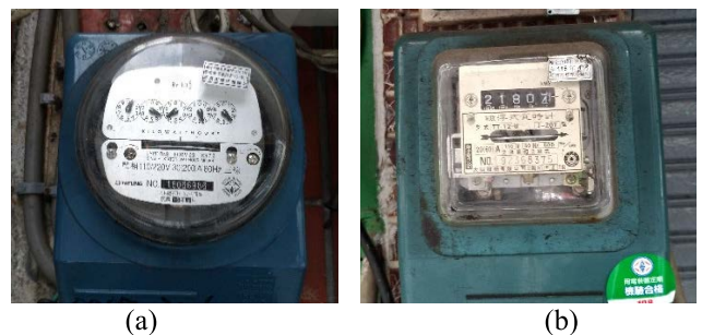
FIGURE 1. Two types of electricity meters. (a) Dial meter. (b) Cyclometer.
