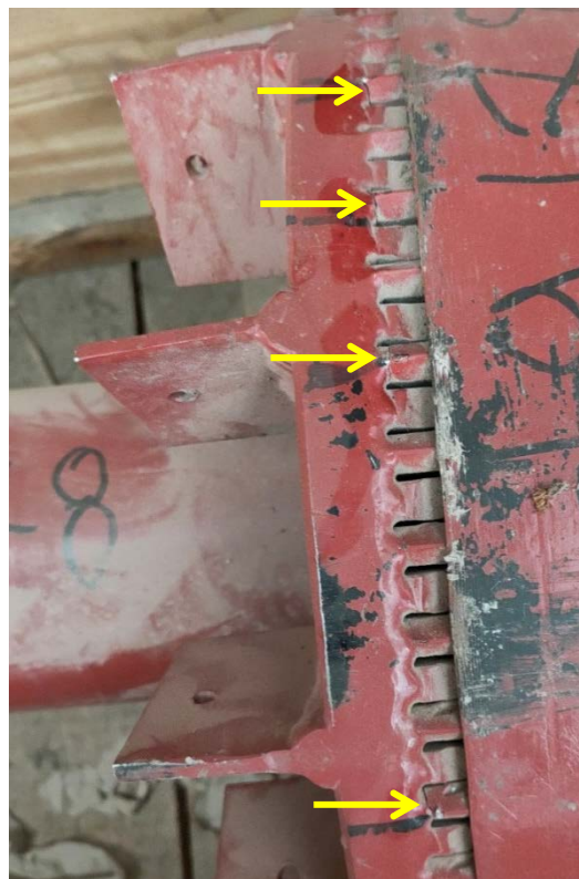
FIGURE 2. Rotor of 380 kW, 6.6 kV motor with multiple broken bars marked with yellow-colored arrows (the photo is taken by the authors).
