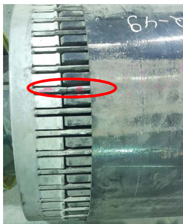
FIGURE 1. Rotor of 460 kW, 6.6 kV motor with one broken bar marked with red color (the photo is taken by the authors).
