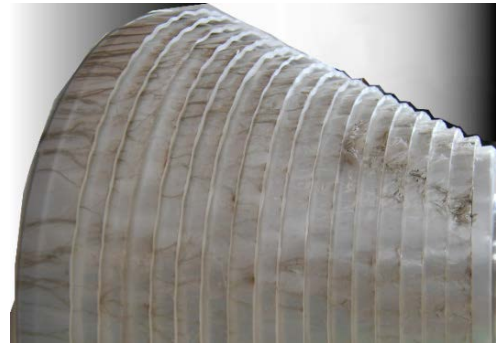
FIGURE 2. Flashover traces on the conical surface of the peaking capacitor.
