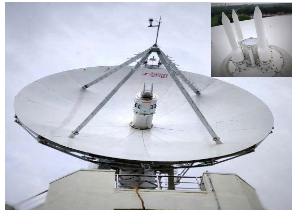
FIGURE 11. Installed composite feed in the reflector.
