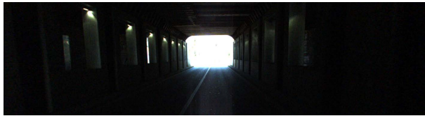
(b) Tunnel passage in sequence 10_02.
