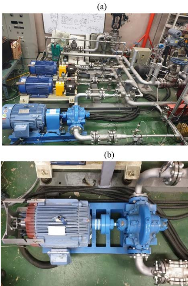
FIGURE 3. (a) Flow loop for the experimental data and (b) A centrifugal pump for the experimental data.
