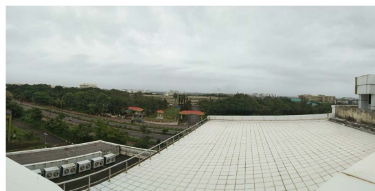
FIGURE 15. Panoramic view from location B focusing towards building A. This building is marked as site 2 antenna 2 in the cell site area map.
