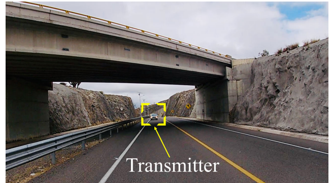
FIGURE 10. Section of the road with steep mountains on both sides and an under bridge pass (Receiver camera).
