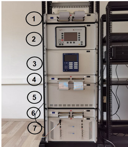
FIGURE 6. Microgrid Typhoon-HIL testbed.
