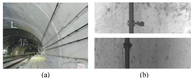
FIGURE 1. The samples of leaky cable fixture. (a) Tunnel and leaky. (b) Faulty cable fixture and normal cable fixture.
