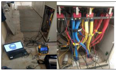
FIGURE 3. Systematic energy auditing phase using class 'A' Instrument.
