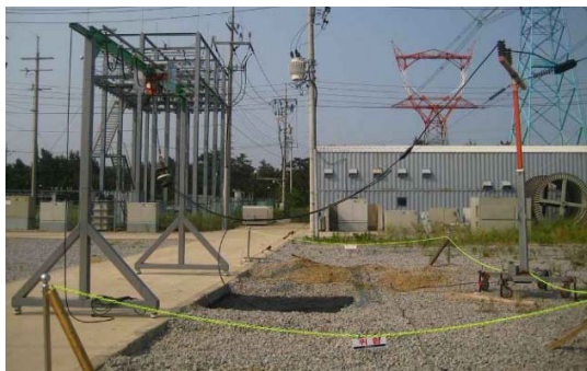
(a) Installation of equipment for experiments
