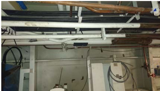
FIGURE 13. Testing of tag reading angles inside the OPV.
