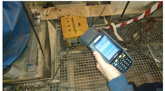
FIGURE 14. Tag reading in an area of very high density of metallic objects.
