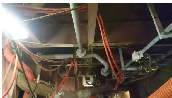
FIGURE 4. Mounted pipes on the ship ceiling.
