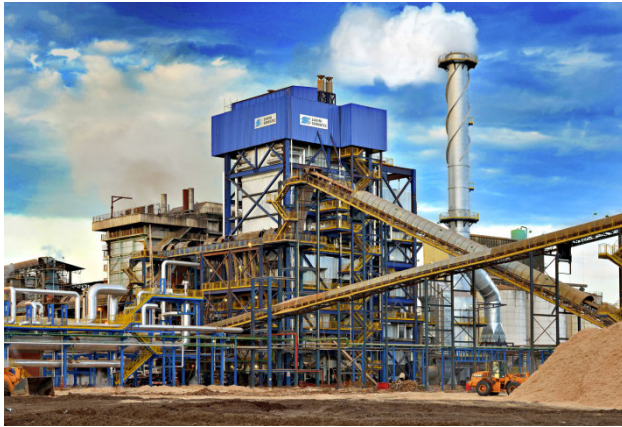
FIGURE 1. View of a bagasse-fired boiler.
