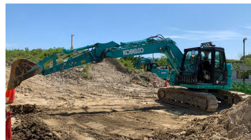
FIGURE 18. Actual image of teleoperated hydraulic excavator in experiment.
