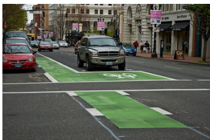
FIGURE 10. Schematic diagram of the bicycle stop line and pre-stationed motor vehicle stop line at intersection.
