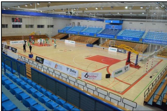
FIGURE 1. Real scenario under analysis: Sport pavilion located at the public university of navarre.
