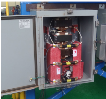
FIGURE 3. The three-phase inductors at the surface: Real choke.
