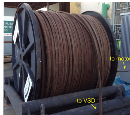
FIGURE 6. ESP components: Three-phase power cable.
