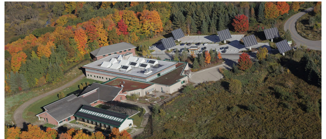
FIGURE 18. Aerial shot of the Kortright Centre Microgrid, which shows the PV system and smart homes on the west side of the microgrid.
