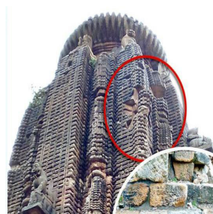
FIGURE 5. Lightning Strikes in (a) Jameswar and (b) Nilamdhhab Temples respectively.
