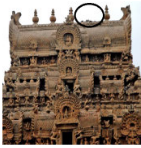
FIGURE 1. Brihadishvara Temple – Lightning Strike shattered the spire atop Rajarajan Tower (Gopuram) in 2010.
