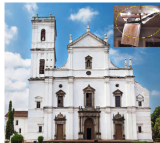
FIGURE 6. Damaged roof and gables due to lightning strikes in Se Cathedral and Basilica of Bom Churches at Goa during 2015 and 2016 respectively.
