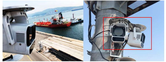
FIGURE 8. Experimental setup with two AVMS sensor modules. The AVMS sensor modules are currently installed at Ulsan port in Korea and being pilot tested.
