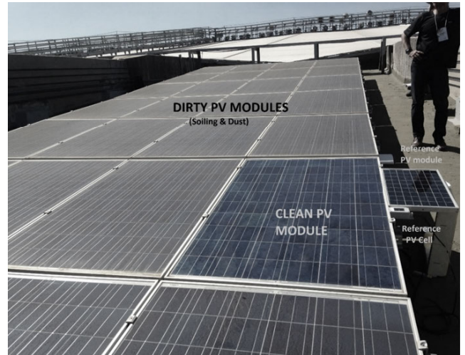
FIGURE 7. Cleaning of the PV module.
