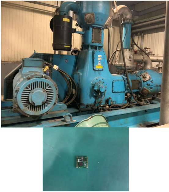
FIGURE 6. Vibration sensors in different locations in air compressor.
