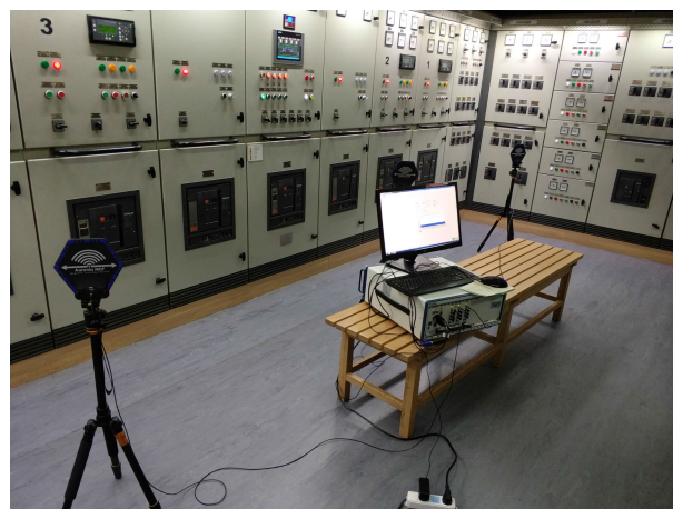
FIGURE 8. Photograph of a testing site inside the cruise ship.
