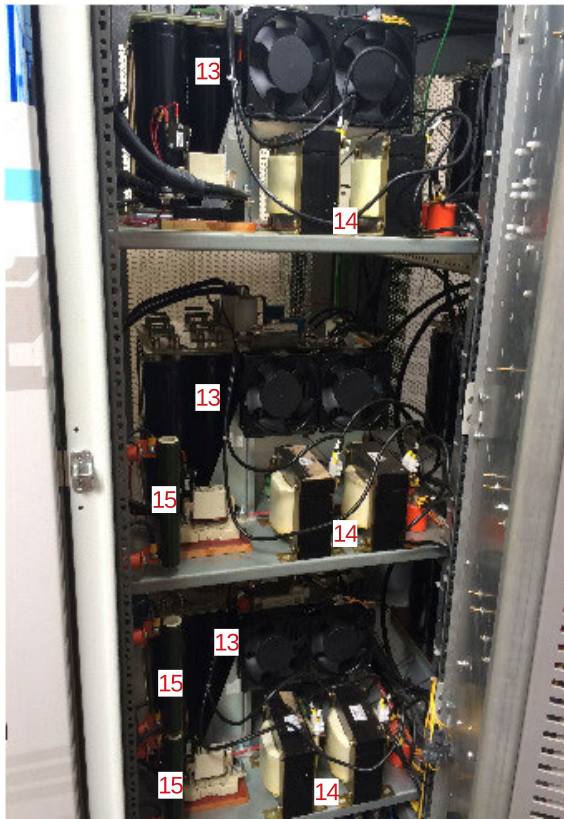
FIGURE 15. Power subsystem (of one phase).
